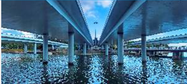
Smart Treatment for Water
